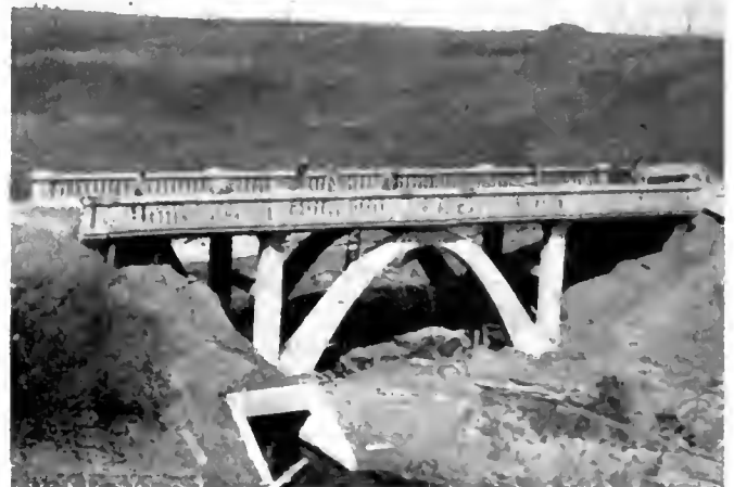
The bridge over McKinnon's Ravine is a two-ribbed open spandrel arch of reinforced concrete
